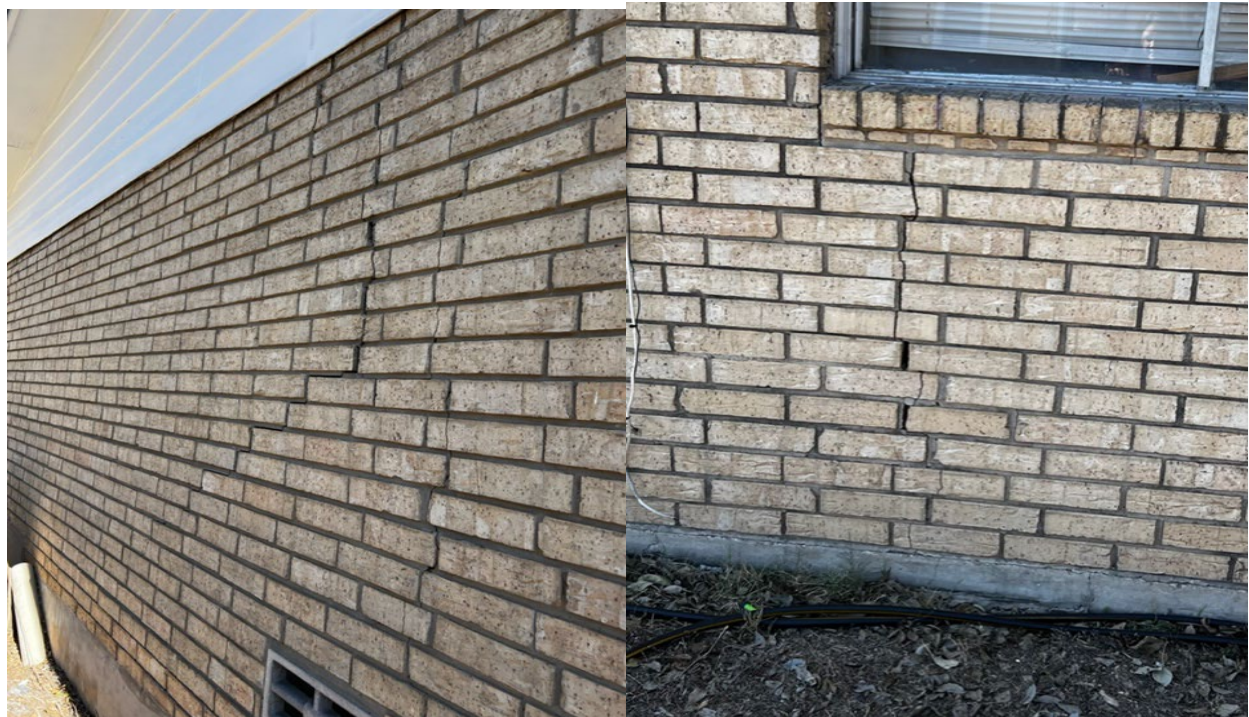
Damage to brick from settling foundation on right and left side of house
